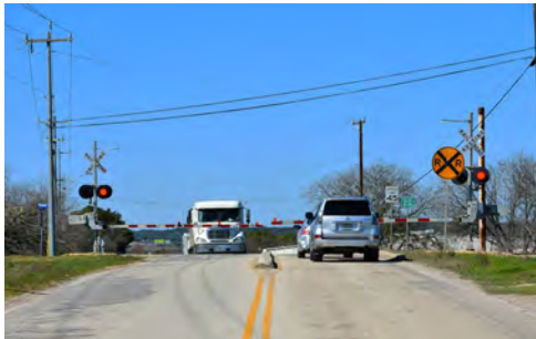
Railroad grade crossing at the intersection of E Evans Road and Wagon Road
